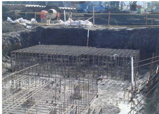
Rebar work for Boiler #1 south side
